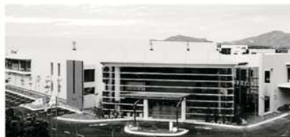
Vitrox plant in Penang
